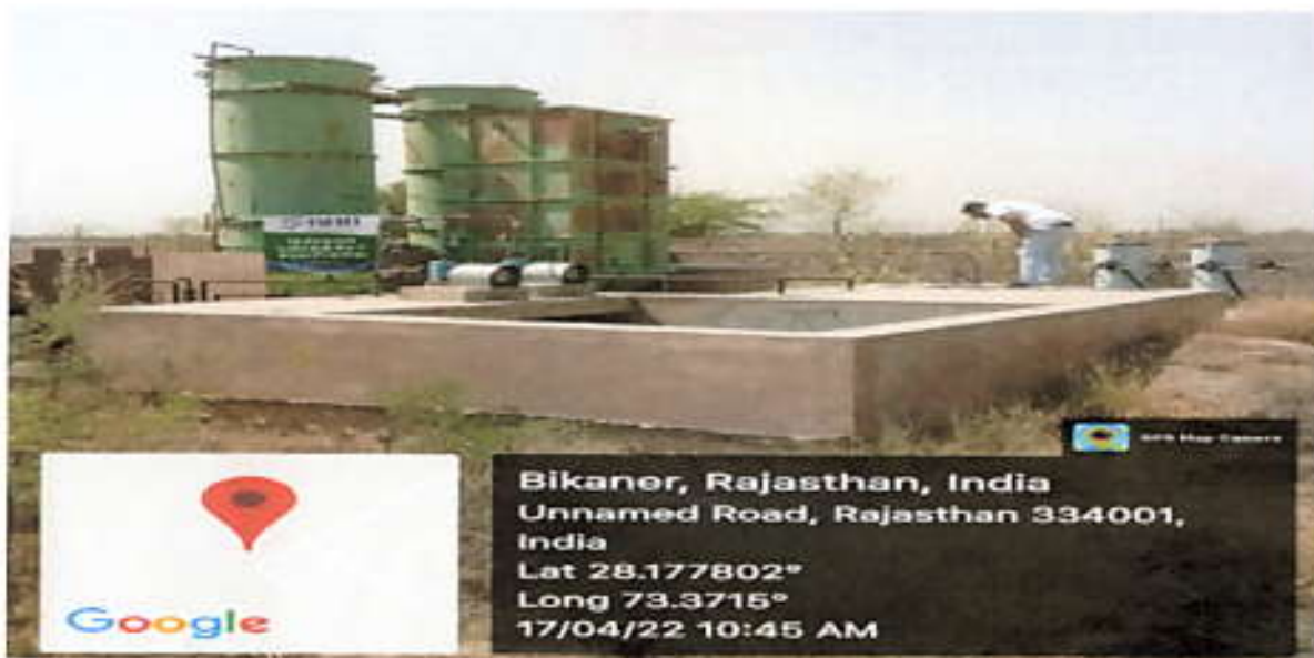
Sewerage treatment Plant of RNBGU
